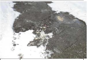
ASPHALT NEEDING SEALCOAT AND FUTURE MILL AND #72: **OVERLAY**
