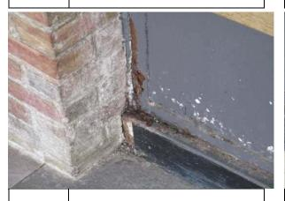
**RUSTING CURTAIN WALL** #11: PANEL AND EFFLORESCENCE
