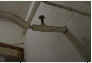
PIPE INSULATION WITH #6: POSSIBLE ASBESTOS
