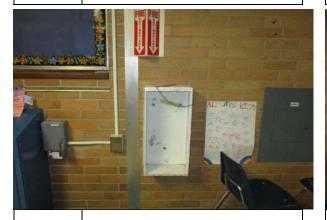
FIRE EXTINGUISHER CABINET, #53: MISSING COVER AND FIRE **EXTINGUISHER**
