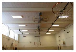
SOUND DAMPENING CEILING #23: TILES POTENTIAL ASBESTOS MATERIAL (ACM)
