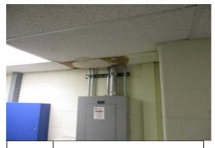
SUSPENDED ACOUSTICAL TILE #19: (ACT) WITH SIGNS OF ROOF LEAK
