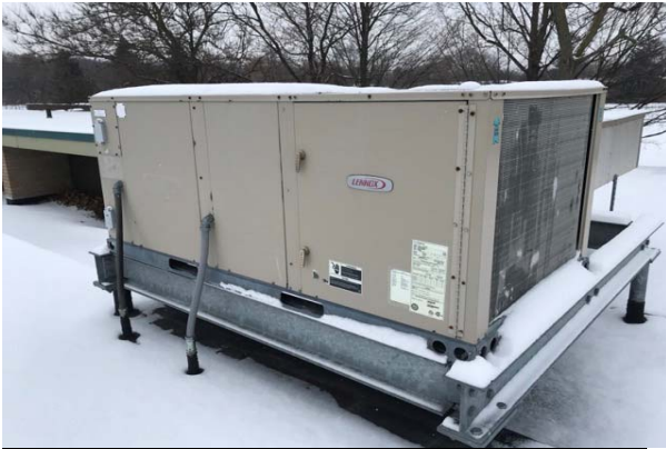
#13: PACKAGED UNIT (RTU),
