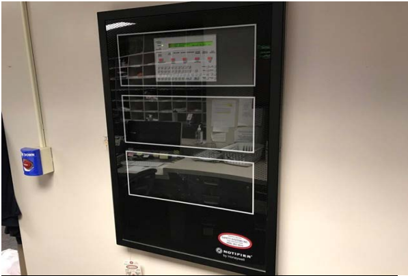
#43: FIRE ALARM CONTROL PANEL
